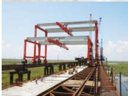
*The new bridge on the LA 1 Highway is being constructed from the top down to minimize impact on the coastal wetlands areas over which the bridge is being constructed.*
