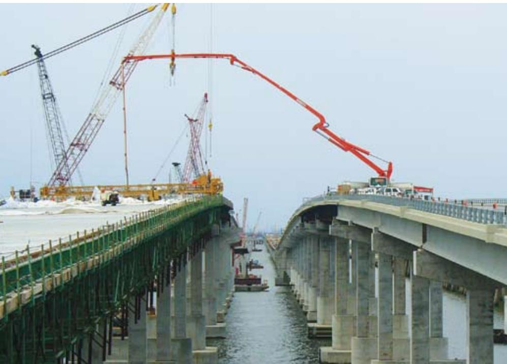
*The I-10 Twin Spans as they approach the main channel. The goals for these replacement structures include better storm protection, safe accommodation of six traffic lanes, enhanced barge collision resistance, and utilization of well-known materials and techniques to provide for low maintenance and long service life.*
