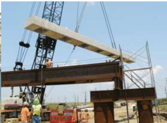
*Nine miles of the LA 1 Highway Bridge are currently being constructed, while an additional 9 miles are being planned and designed. Here a precast concrete pile bent cap is being moved into position for installation.*
