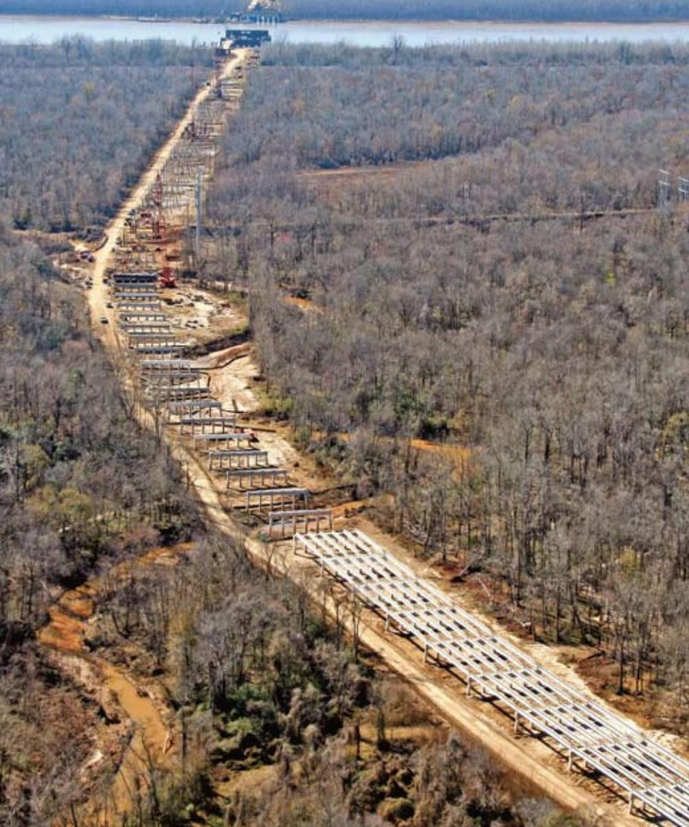
*The 2.44-mile-long John James Audubon Bridge crossing the Mississippi River, to be completed in late 2010, will be the longest cable-stayed bridge in North America. In addition to the precast concrete structure, the project involves seven other bridges featuring Type III AASHTO precast, prestressed concrete girders and 72-in.-deep bulb-tee girders with cast-in-place decks.*
