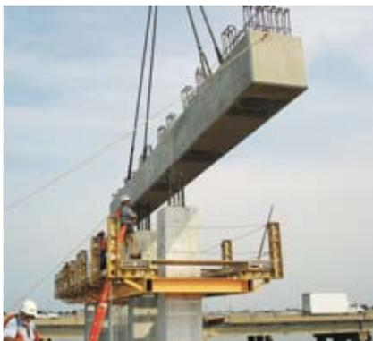
*A precast concrete bent cap being set on precast concrete piles for the I-10 Twin Spans Bridges over Lake Pontchartrain.*
