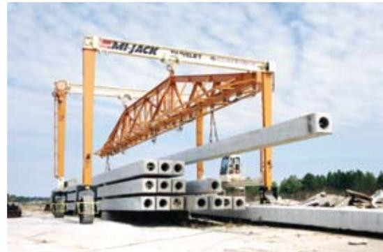
*Twenty-four-inch- and 30-in.-square piles were cast with high-strength concrete permitting longer individual lengths.*
