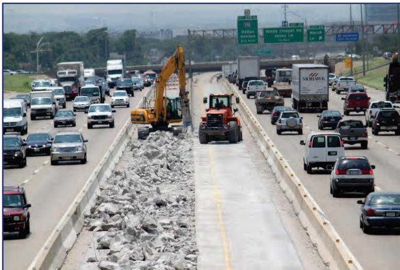
One of the most challenging aspects of the road design was the maintenance of traffic plan. Complex traffic maintenance plans to meet the stringent contract criteria that all lanes must remain in service for the duration of the construction were developed in cooperation with the contractor. All lanes remained open while completing the 30 foot deep excavation down the center of the existing highway.
