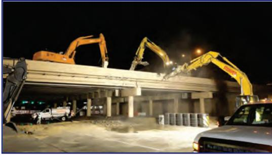
equipment to verify the structures could safely support the equipment during the staged removal. JSE considered not only the plan information, but looked at inspection reports to determine if additional consideration must be given to deteriorated components. In the event where traffic was maintained under structures that were being demolished, JSE designed protective sheeting to further ensure safety to the travelling public.
