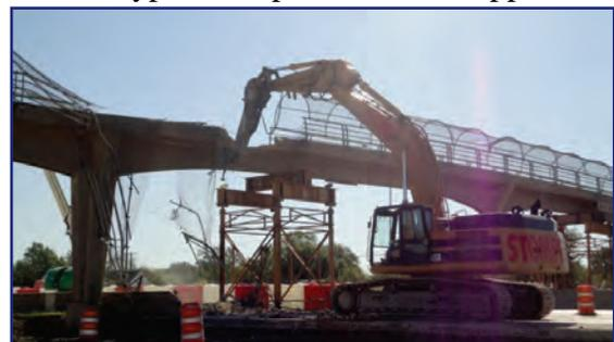
The analysis performed on some of the structures concluded that in order to maintain stability during demolition, temporary shoring would be required to support the structure. When this was the case, JSE either provided the anticipated shoring loads for use with standard towers or in unique cases, JSE designed a shoring system for the contractor to use.
