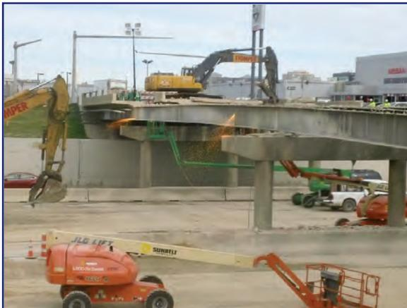
Prior to various construction operations taking place, demolition of the existing structures in this project had to take place. JSE prepared the demolition analysis for the existing bridge structures to be removed. Working closely with the contractor, JSE developed and produced the controlled, staged removal demolition plans for all the structures.
