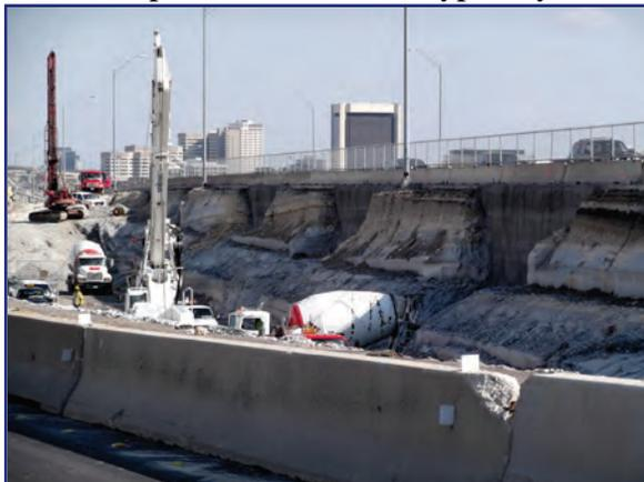
relied on a combination of skin friction and end bearing to achieve capacity. If geometry dictated, group effects were also considered in their design. This foundation type was selected based on the soil type (clays) and close proximity to rock.
